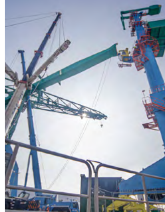
RIKON process includes crane design, manufacturing, logistics and installation on premises
